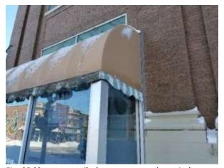
Fig. 05 (Current vestibule canopy cuts thru window location)
