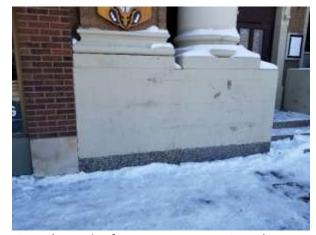
Fig. 03 (Example of Paint on Limestone @ North)
