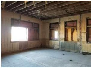
Fig. 01 (Example of several window RO's modified by previous tenant)
