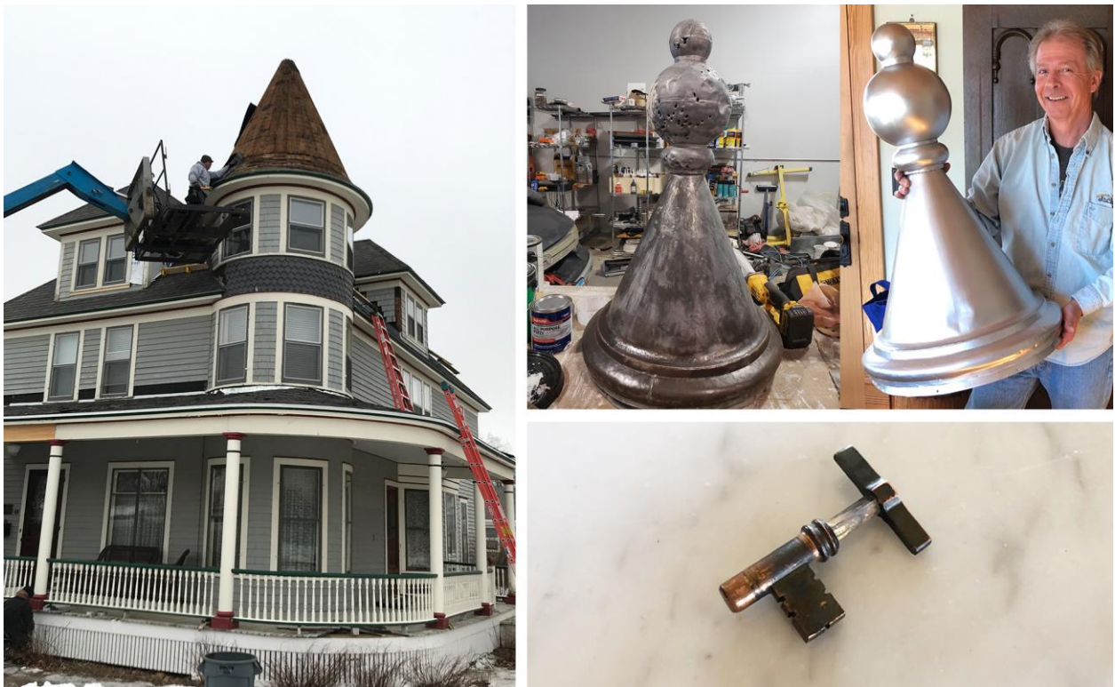
(left) Roofing the turret- photo provided by Thomas Manzer, (top right) Before and after the restoration of the finial- photos provided by Thomas Manzer, (bottom right) A small pocket-door key.
