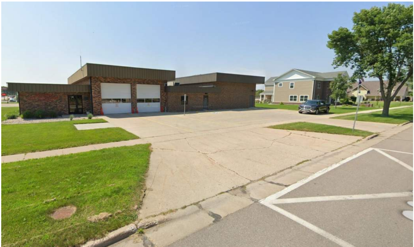
Brookings Fire Department – East Station: approximately 33' apron width and 52' curb cut (with flared approach).
