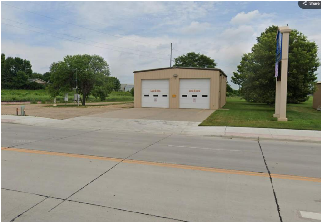
Brookings Fire Department - 22 nd Station; approximately 34' apron and curb cut.
