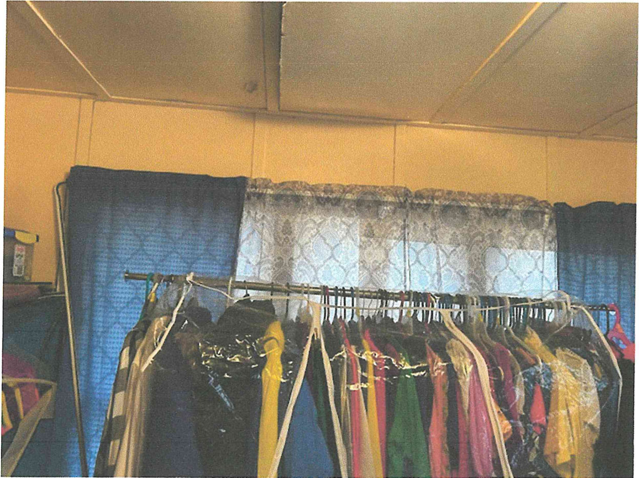
Fig.10. Looking at West interior wall of porch located on main house at 805 4 th Street Note: 3 double -hung windows with wood paneling and ceiling to be replaced insulated
