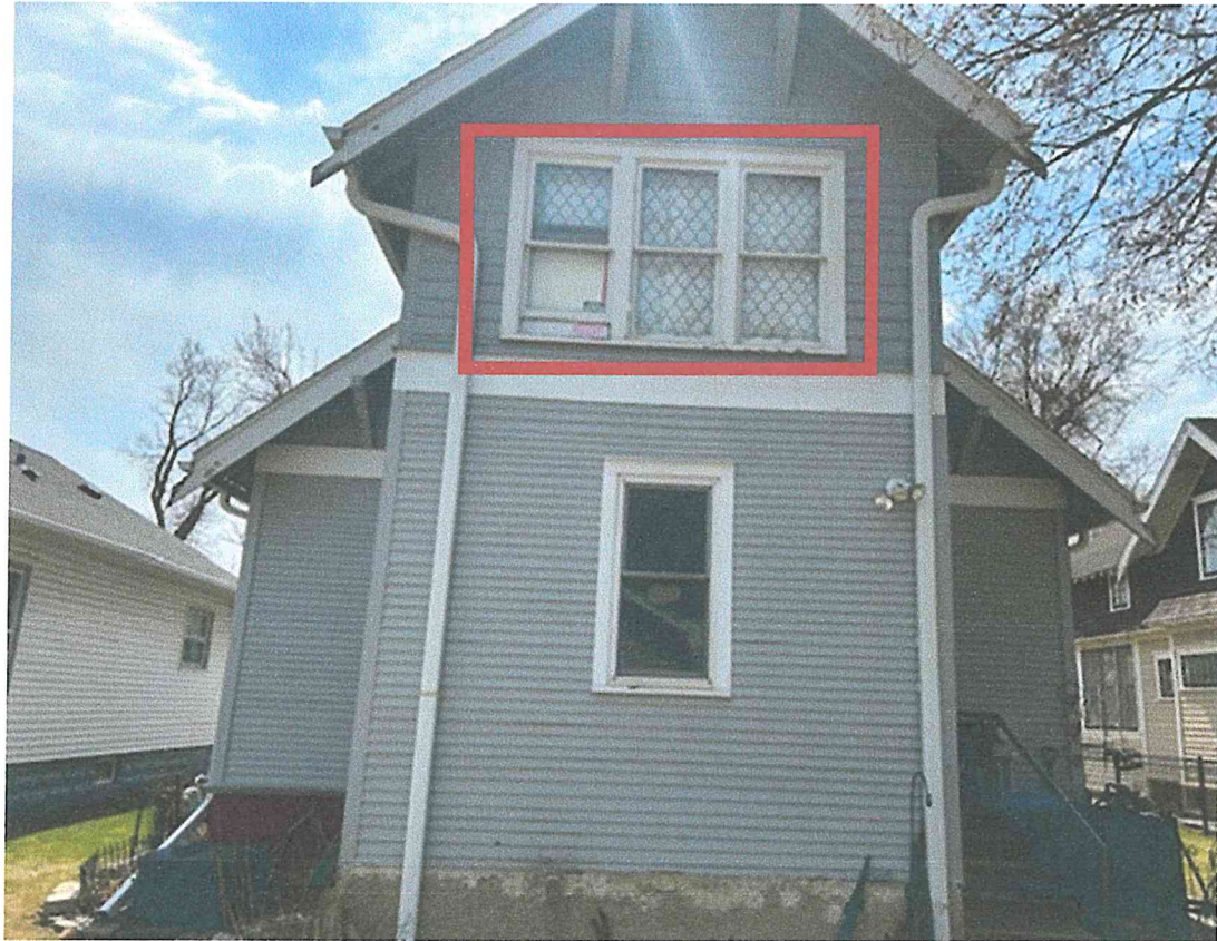
Fig.4. Looking at North exterior wall of porch located on main house at 805 4 th Street Note: 3 double -hung windows on upper level to be replaced.
