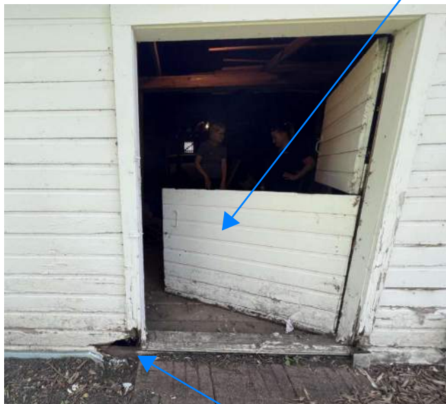
Shift in door frames reflecting settled foundation of east wall.
