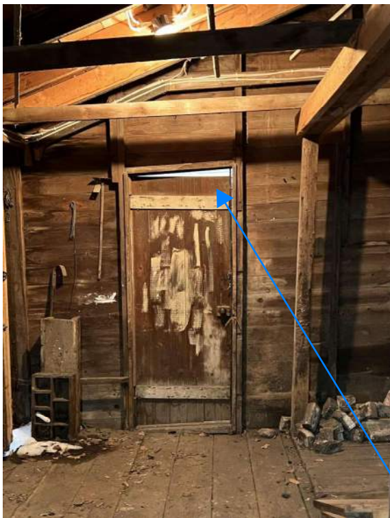
Shift in door frames reflecting settled foundation of east wall.
