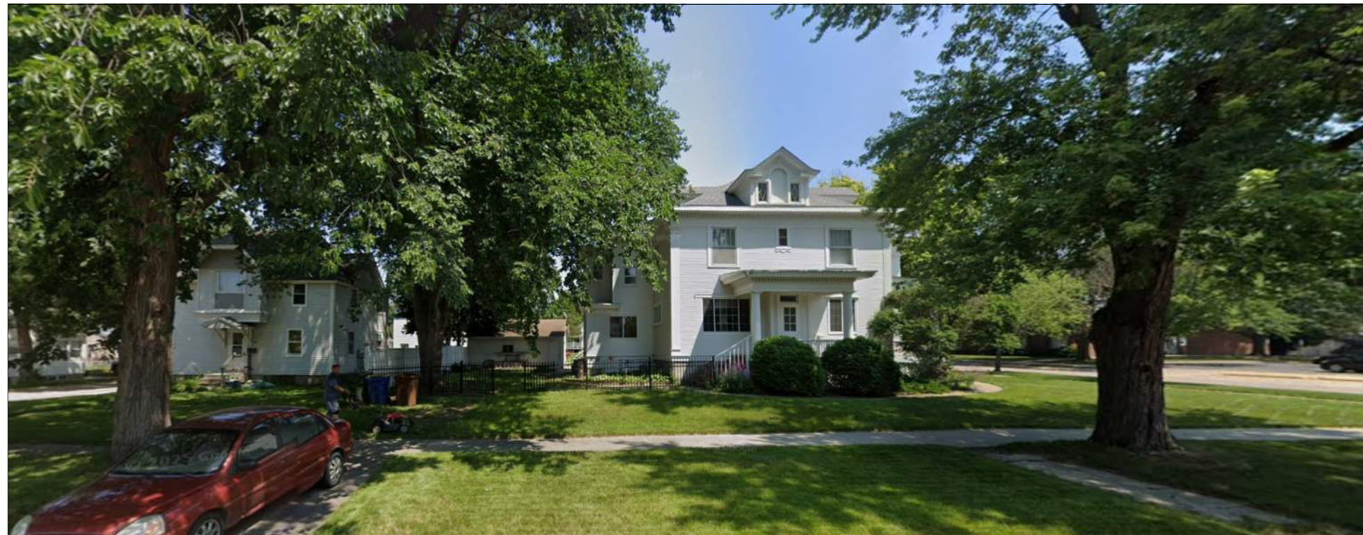
414 9th Avenue and adjacent property and home at 903 4th Street - potential to restore original corner lot
