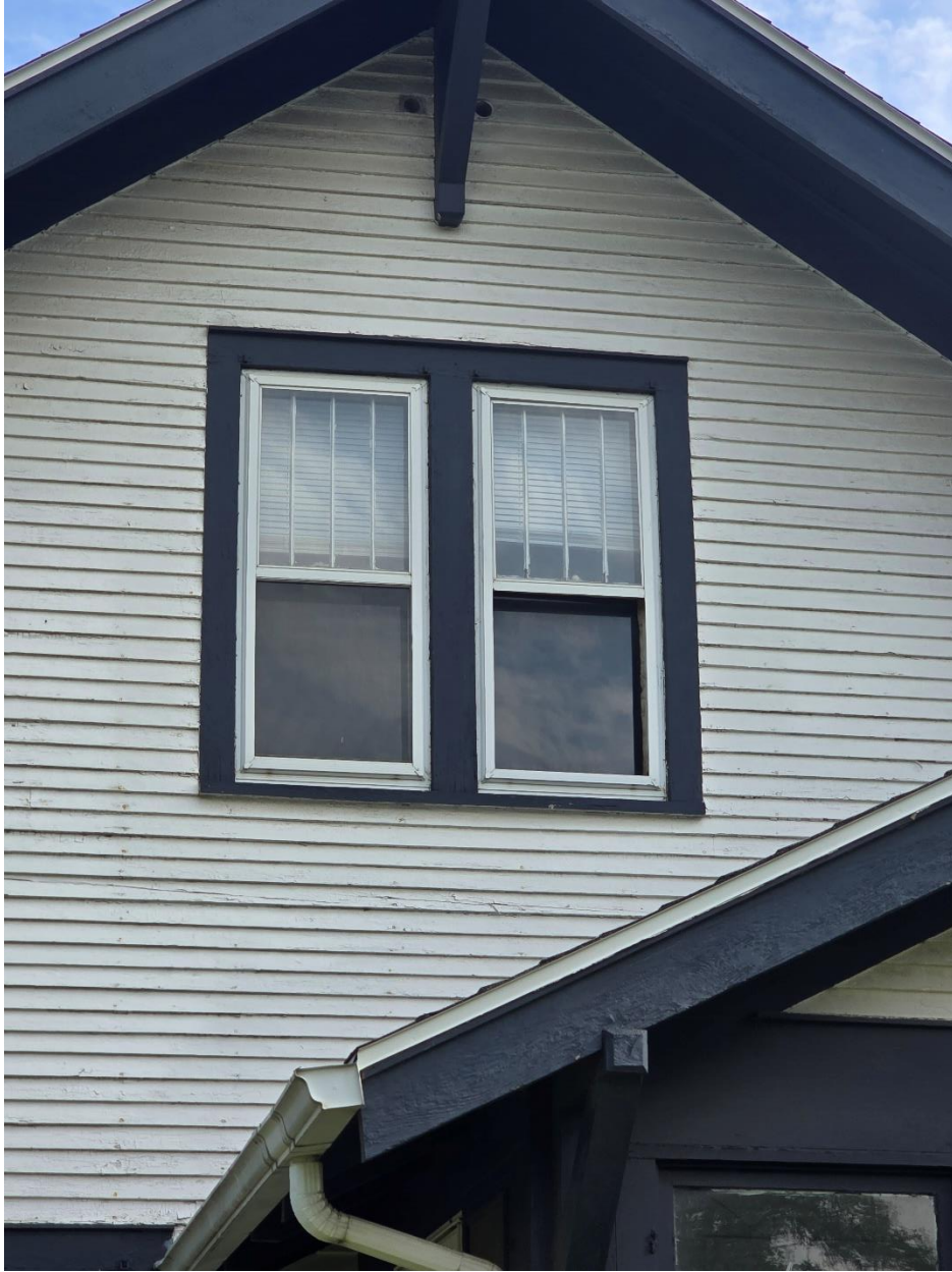
Figure 2: South Window to be replaced
