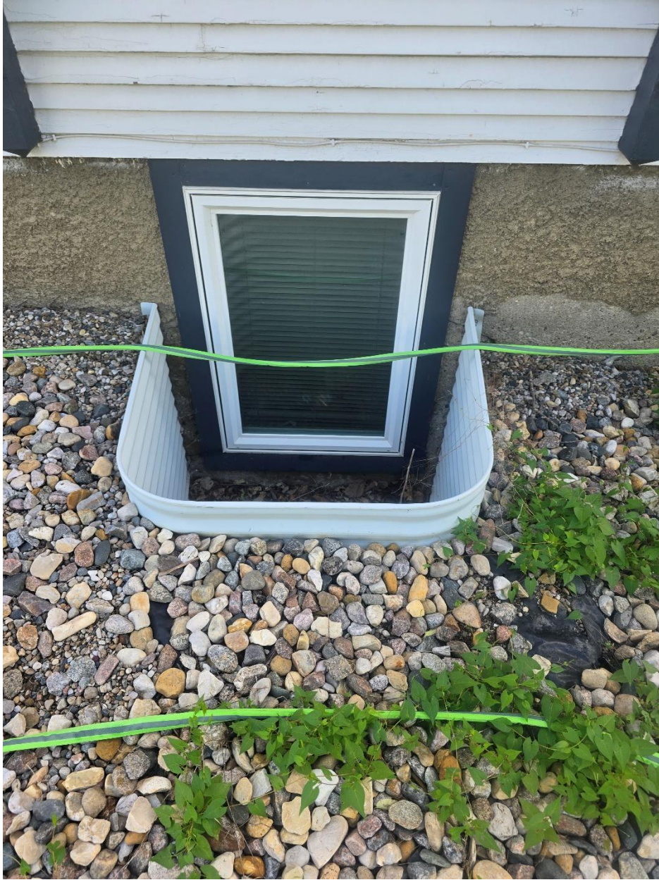
Figure 5: Existing Vinyl Window
