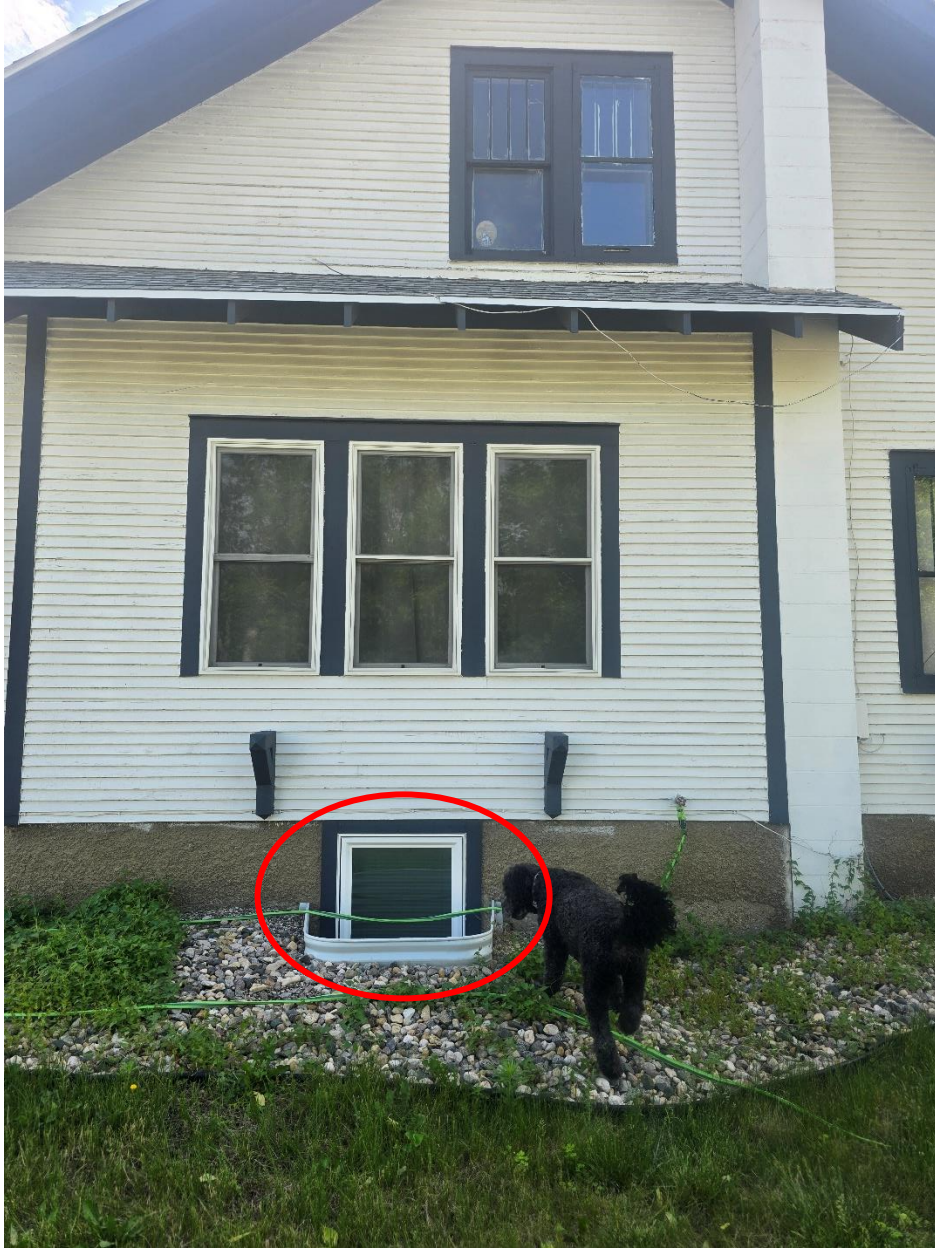
Figure 4: Existing Vinyl Window
