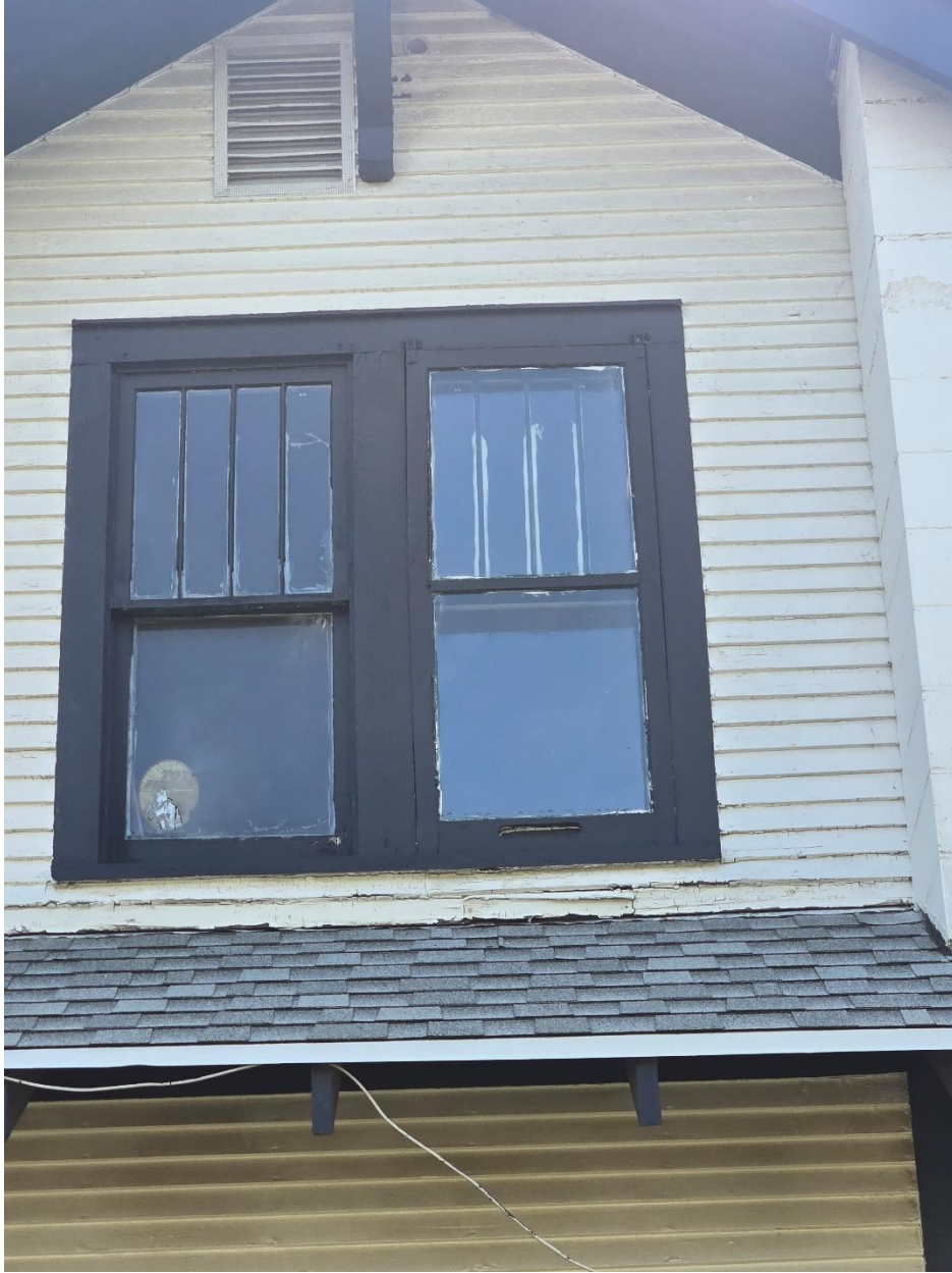
Figure 7: West Windows to be Replaced
