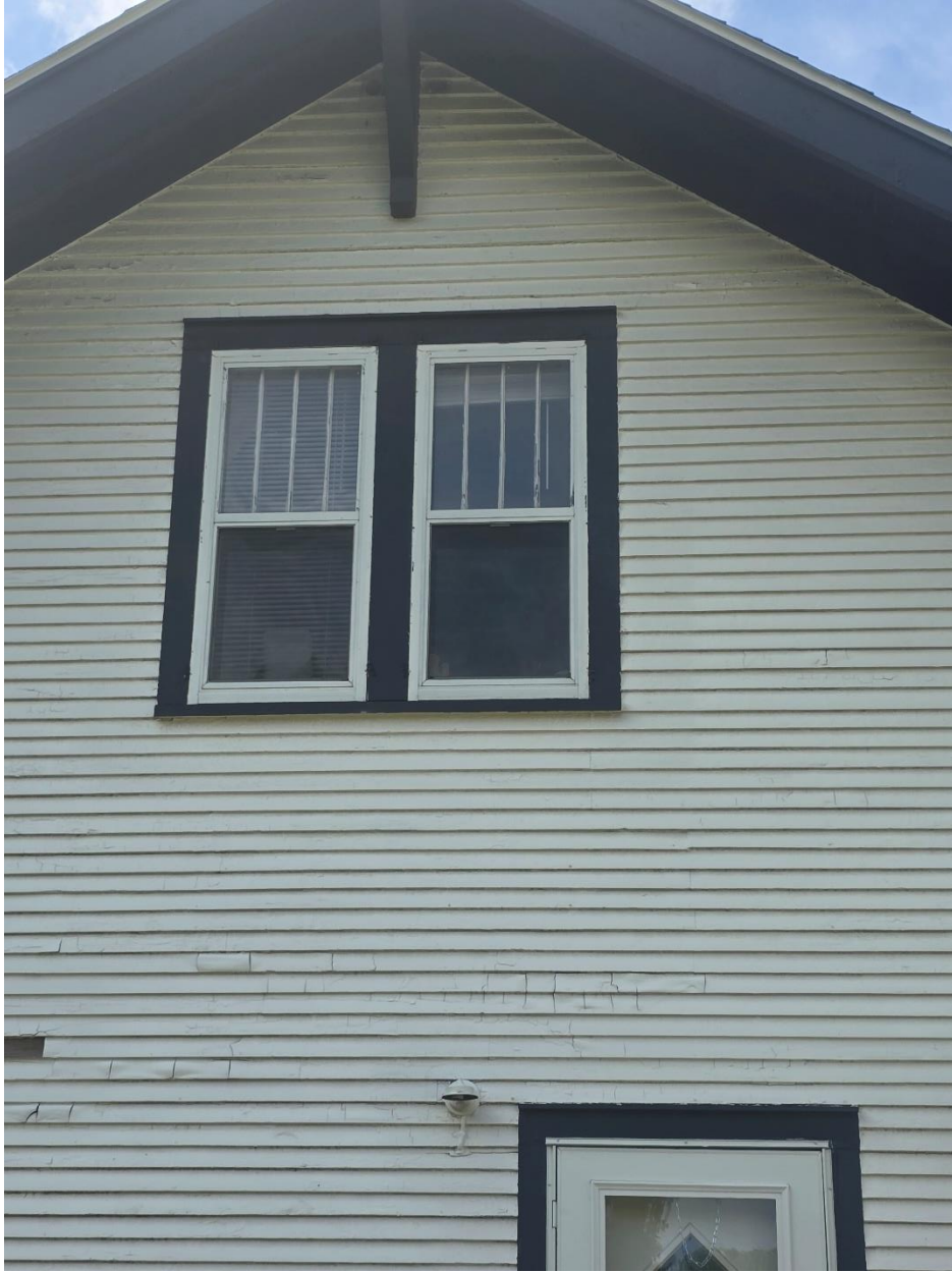
Figure 3: North Window to be replaced
