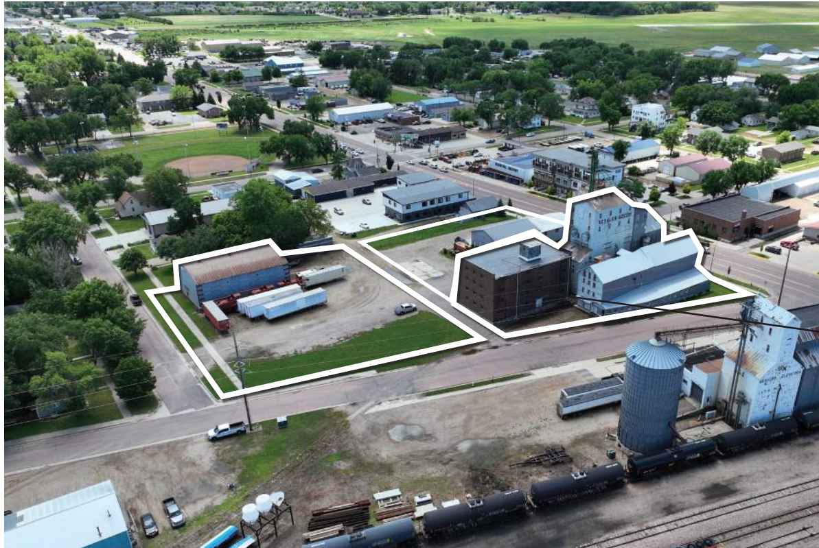
Aerial view looking southwest overlooking the Sexauer Seeds Elevator and nearby property. These sites are subject-to-change and offer development opportunities near Downtown.
