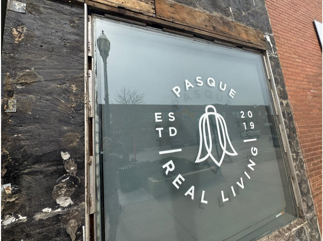
Figure 9: South side storefront
