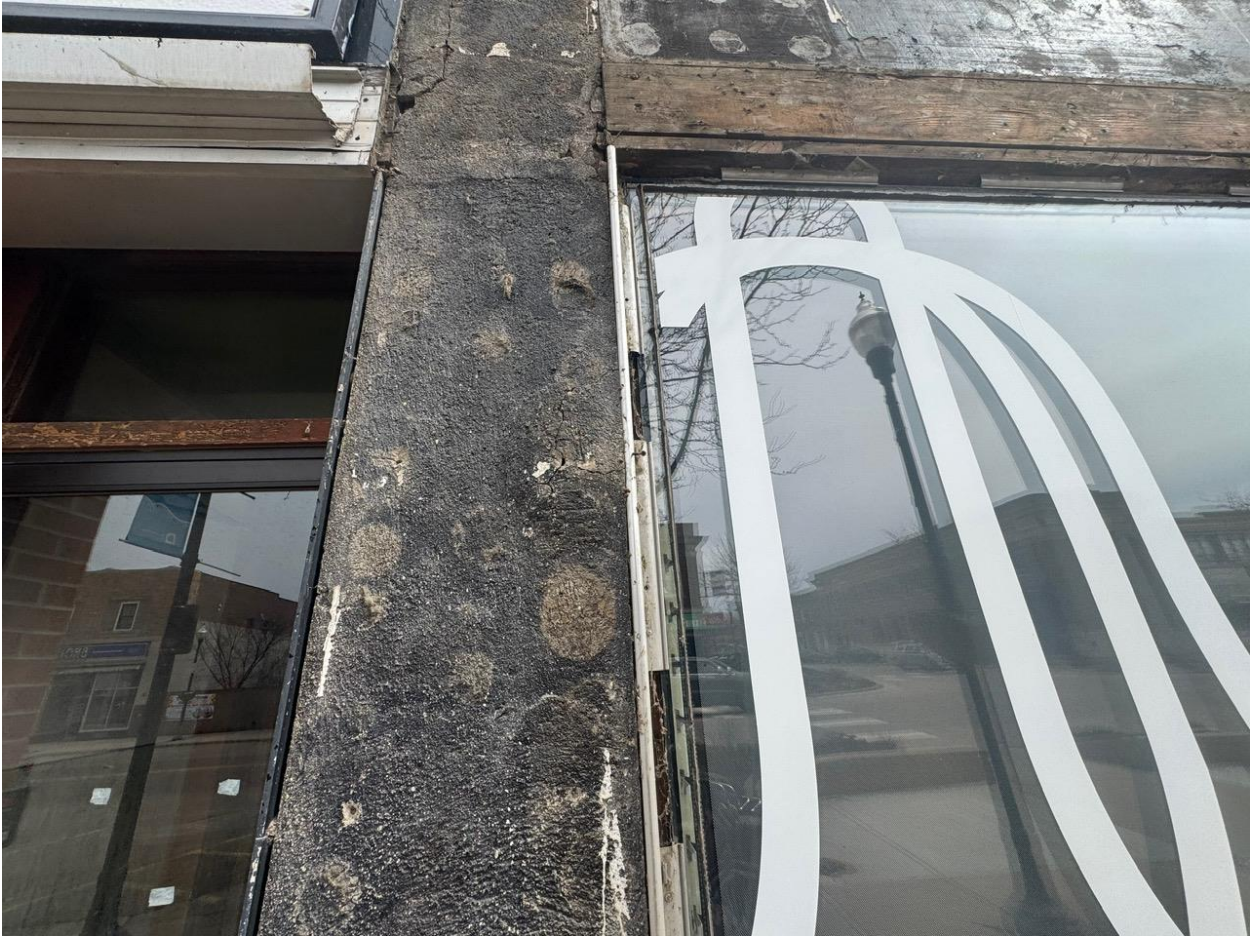
Figure 4: Close up storefront
