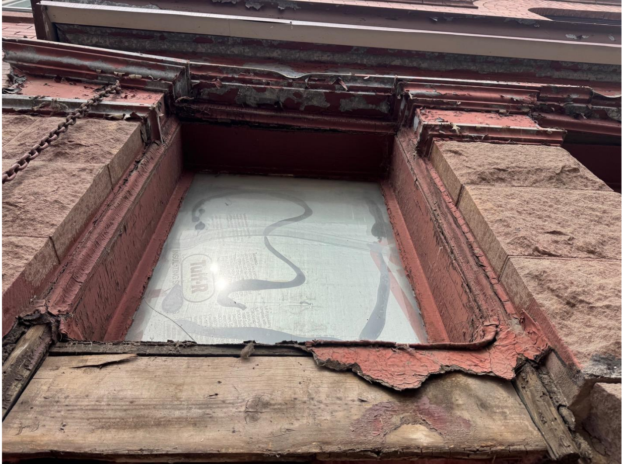
Figure 11: Window revealed under wood siding
