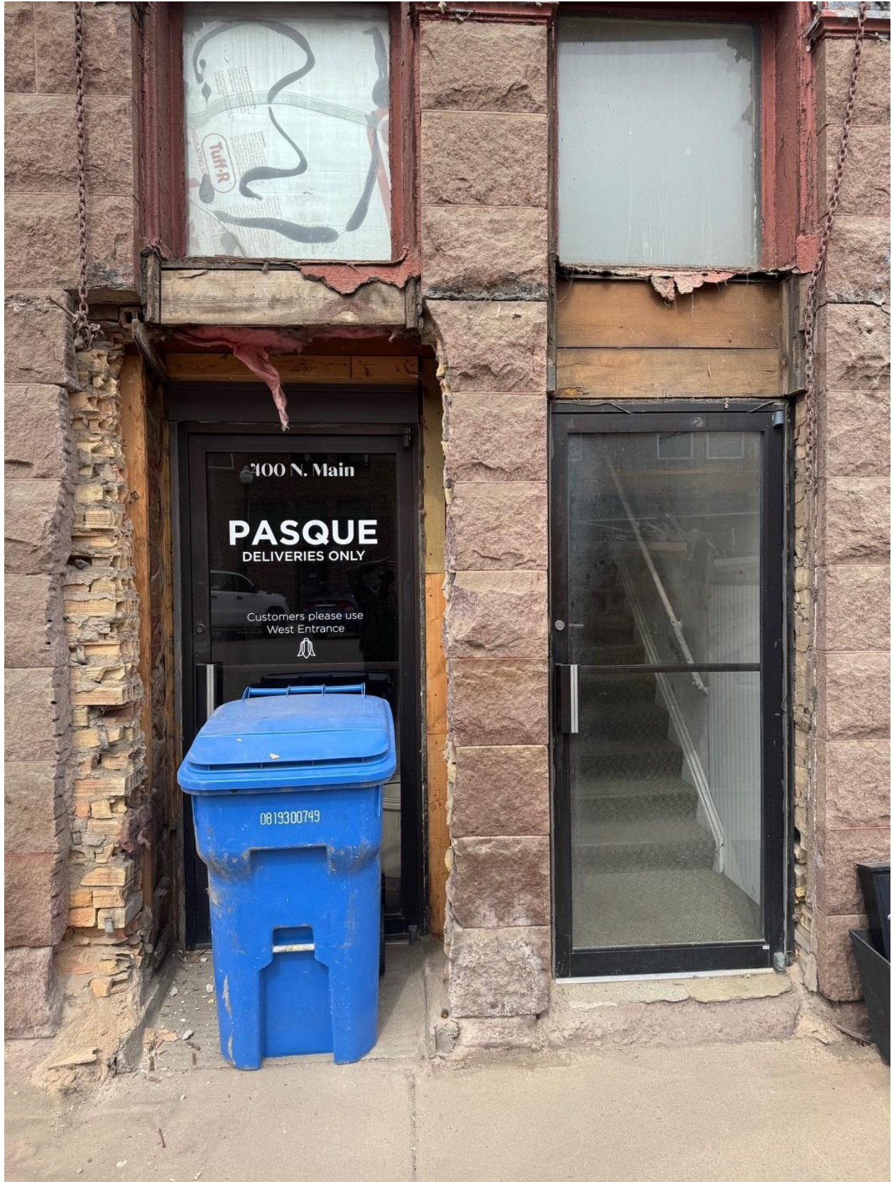
Figure 12: South side wood siding removed
