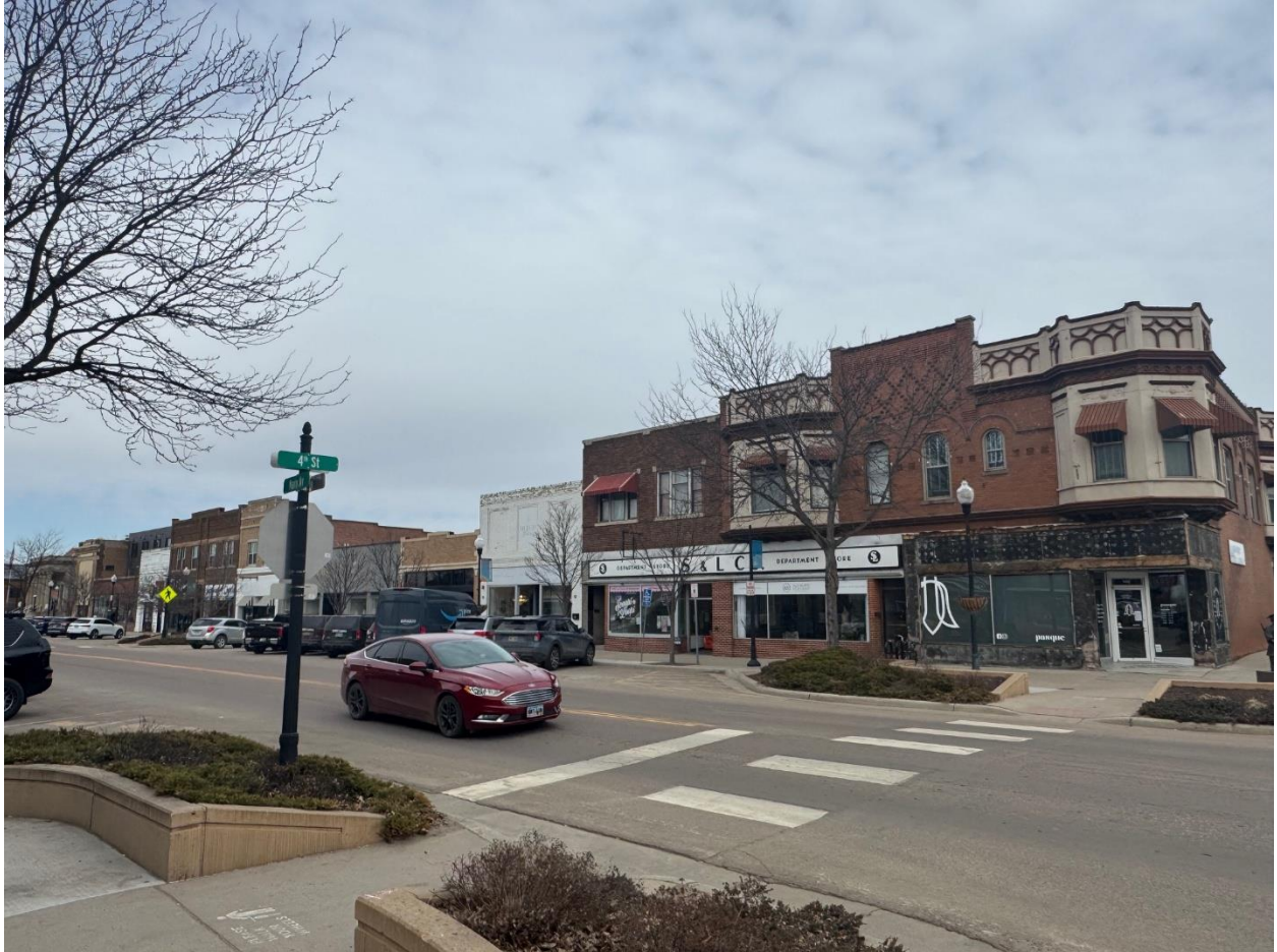
Figure 16: south view of building
