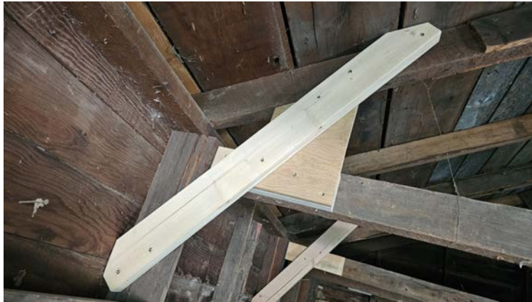
Cracked wall studs with temporary bracing
