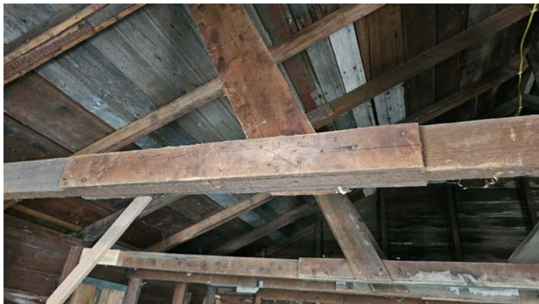
Sagging spliced Rafters and roof line
