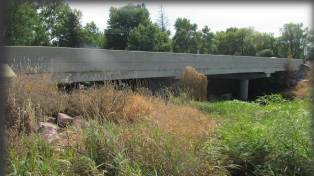
Str. No. 06-170-147 99.5' 3-Span Continuous Concrete Bridge Built in 1987
