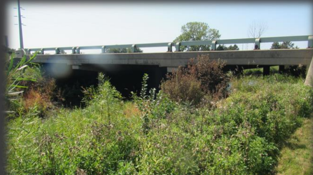
Str. No. 06-170-149 67.0' 3-Span Continuous Concrete Bridge Built in 1968
